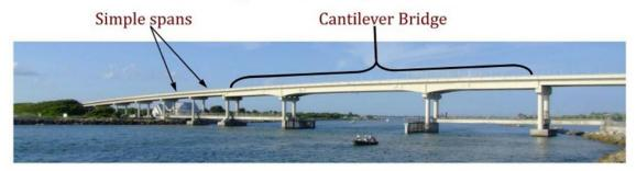
Year of construction: 1965, Total length= 472m, Central span = 55m.
