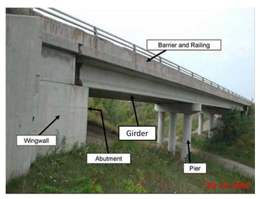
Fig. 8: Different components of a Bridge
