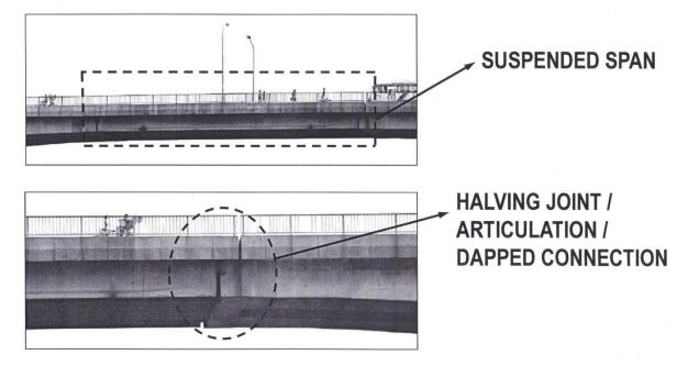
Fig.19: Articulation/ Halving joint
