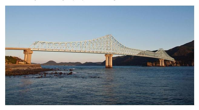
Fig. 3:Truss Bridge – Ikitsuki Bridge, Nagasaki, Japan (Source :online)
